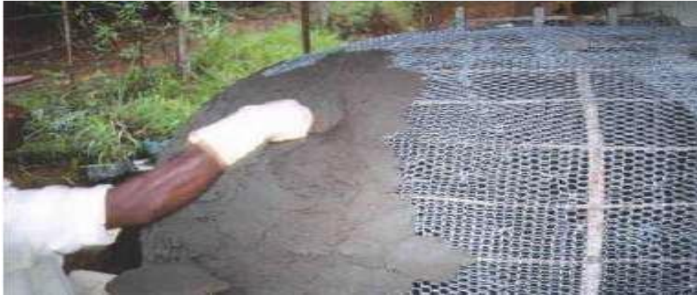
Figure 3-10 Steel mesh reinforcement
