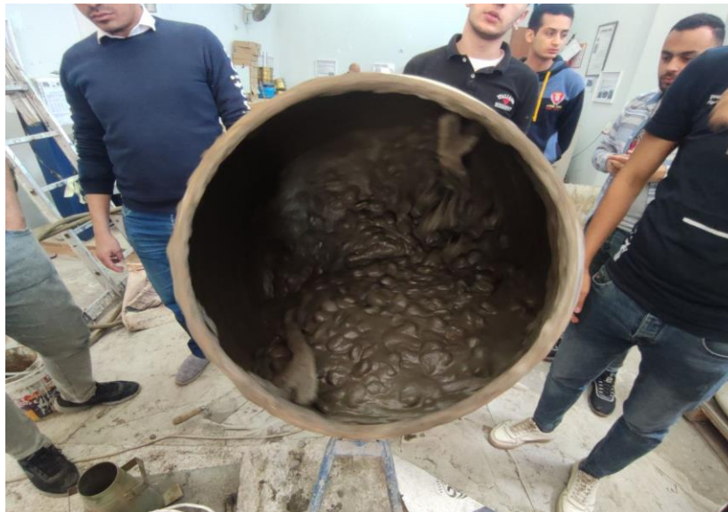
Figure (3-2): Concrete mixing in a batch drum mixer
