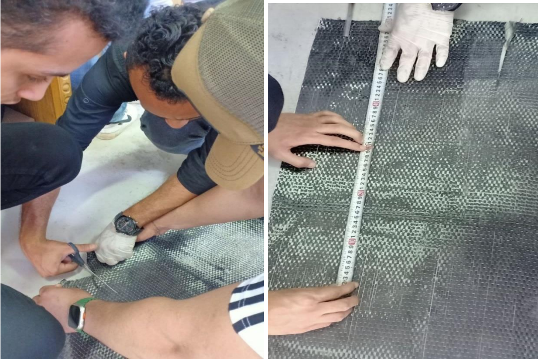
Figure (3-29-b2): Cutting of CFRP sheet to the required dimensions
