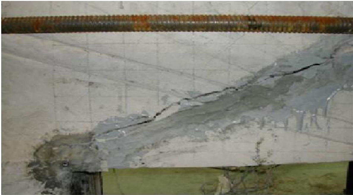
Repair the shear wall
