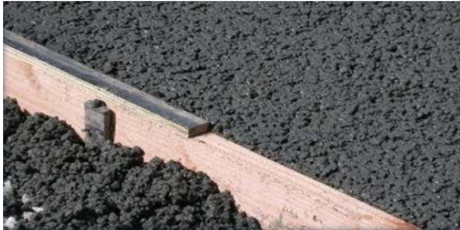
Figure 3-3 No Fines Concrete
